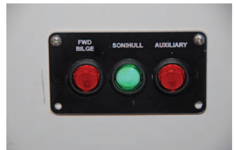
I had run out of breakers at the 12V switch panel, so I had this nifty little panel made up. I placed a 5 amp fuse in the power cable to the control box
